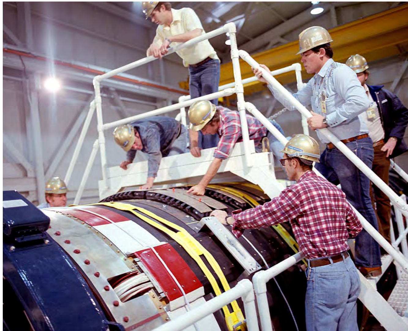
Panel installation takes place on the MGM-118A Peacekeeper weapons system. ©Public Domain.
